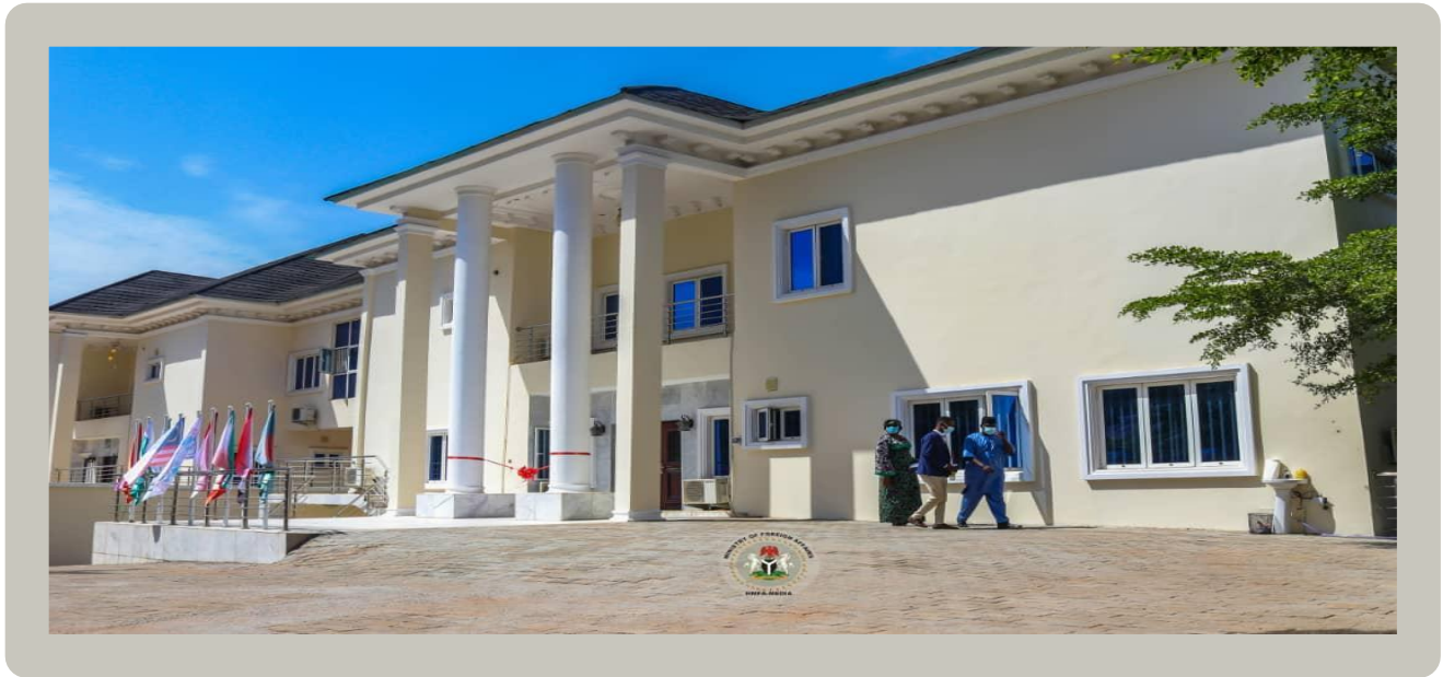
Figure 8: The HSP office premises
